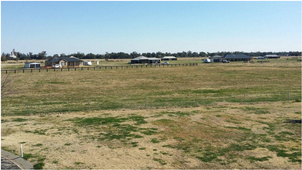
Plate 2: Surrounding Dwellings Constructed within the Flood Prone Land Area
